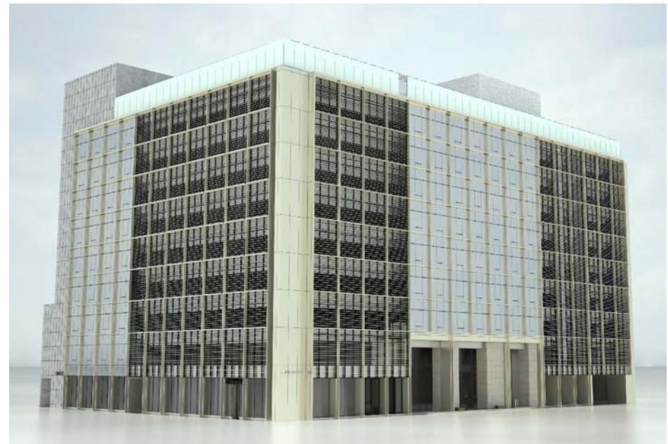
Overview of the Pasona Group Integrated Base
